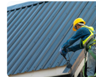
Completing finishing works
