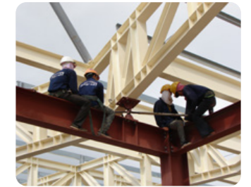
Installing steel frame
