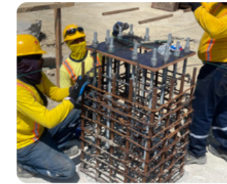
Setting up anchor bolt
