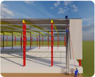
Installing wall sheeting
