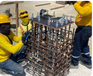
Setting up anchor bolt
