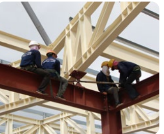
Installing steel frame
