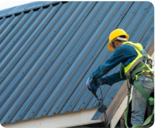
Completing finishing works
